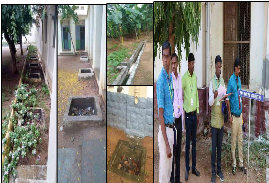
Rainwater harvesting units in St. Xavier's College, Palayamkottai – 627 002, Tamilnadu
